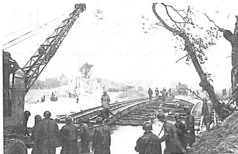
The 16th Engineer Battalion adds steel sections to protect a ponton bridge against the rising waters of the northern Volturno River.
